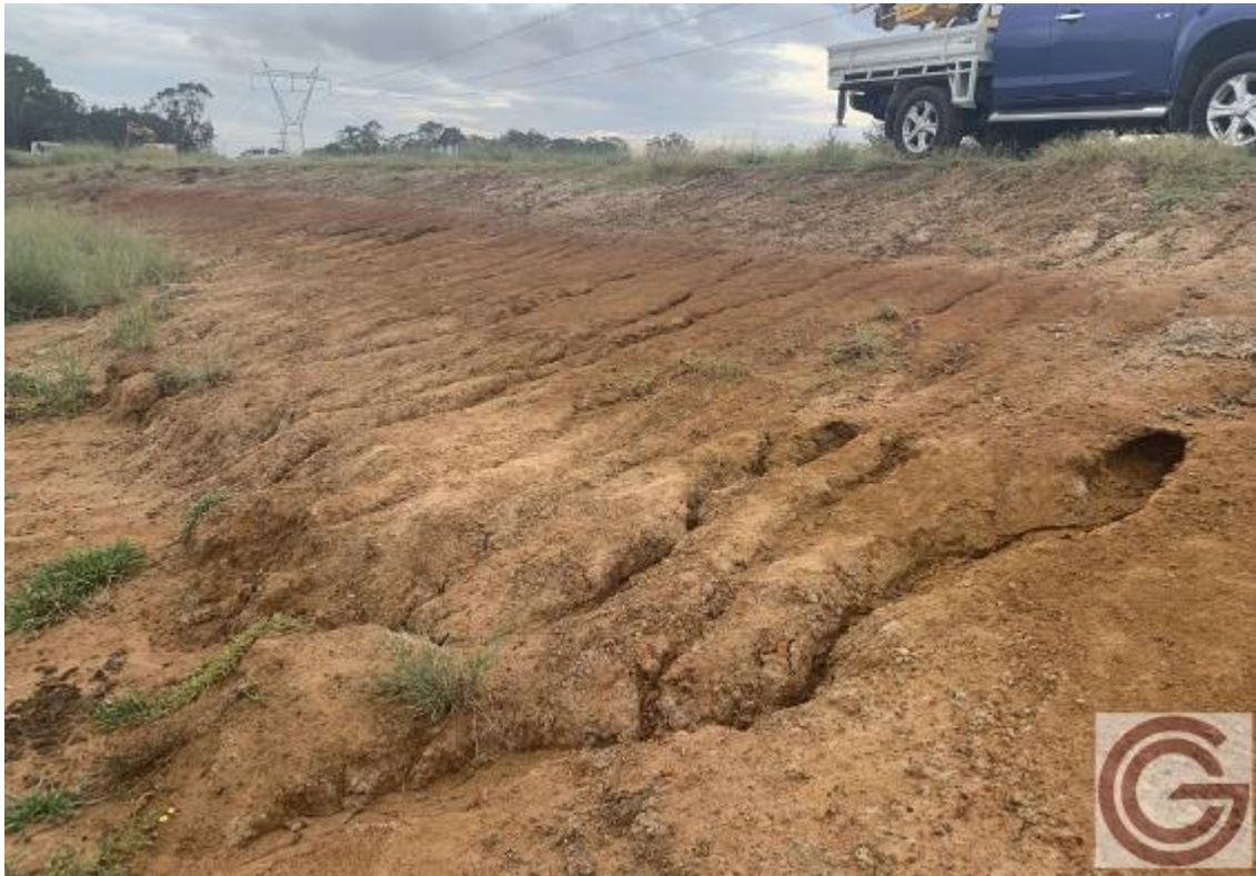
Photo 3: Site view showing signs of soil erosion on the existing dam wall within basin 1
